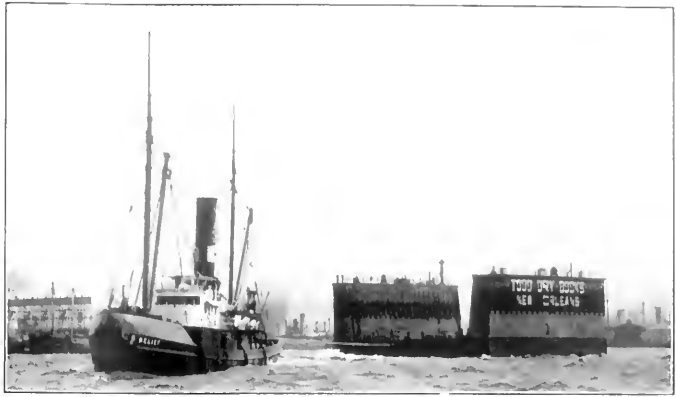
Above is shown the tug Relief towing a 2000-ton section of a floating dry-dock to the plant of the Todd Shipyards Corporation at Algiers, New Orleans from Brooklyn, New York, a distance of 2000 miles. The section is 80 ft. long and 116-ft. wide. The addition of this section will give the plant a dry-docking capacity of 10,000 tons, capable of handling vessels up to 500 ft. in length.
